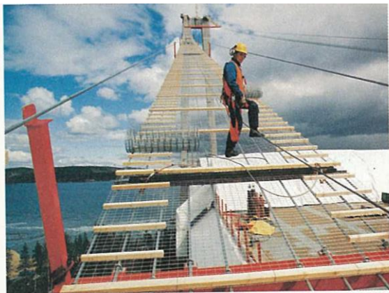
Work on the catwalk, spring 1996
